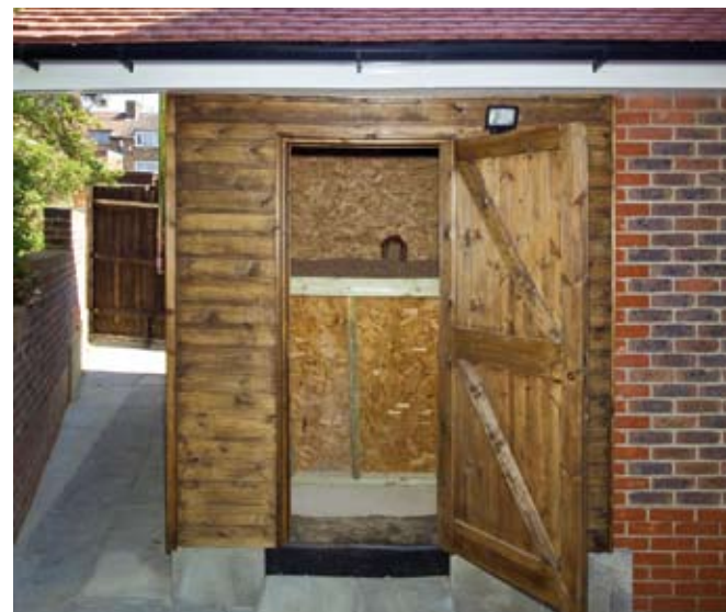
The biomass boiler and store
