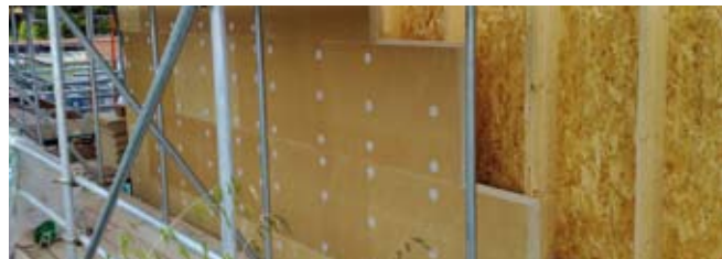
Installation of the cladding
