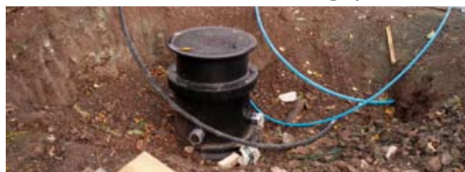
Installation of rainwater harvesting system
