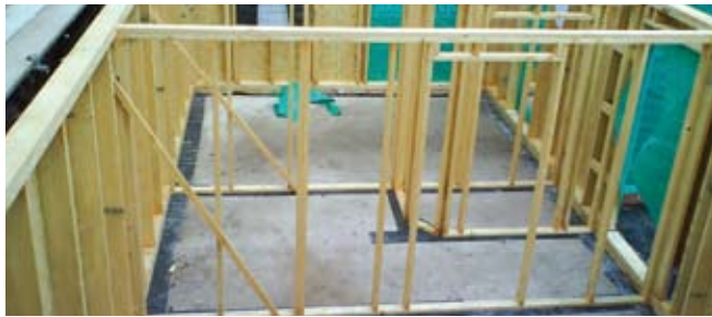
Pre-fabricated timber frame
