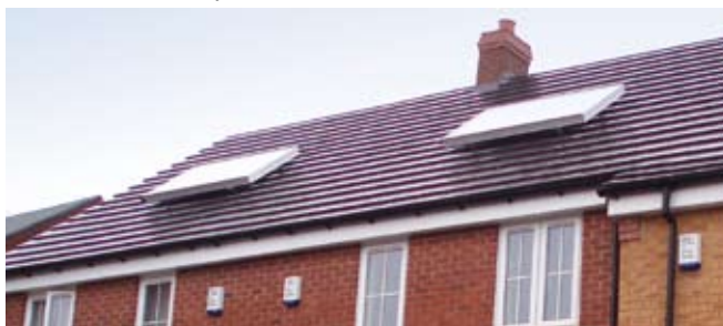
Solar thermal panels on front roof
